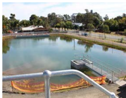
LEFT: SEDIMENTATION LAGOONS UNDER CONSTRUCTION
