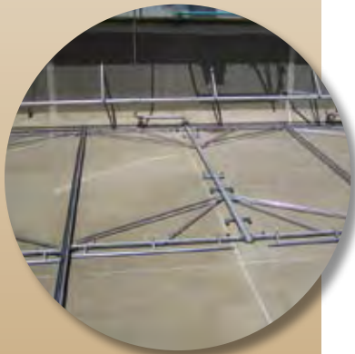
THE EL SOBRANTE WATER TREATMENT PLANT IN OAKLAND, CA INSTALLED 22 MRI HOSELESS CABLE-VAC SYSTEMS.
