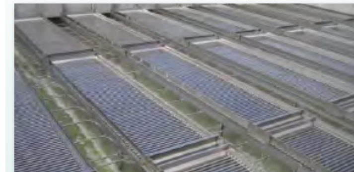
LUGGAGE POINT WWTP (TERTIARY CLARIFICATION)
