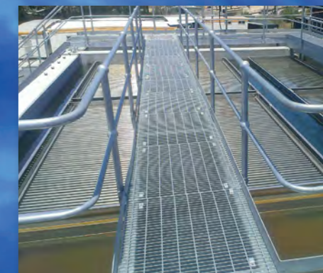
CENTENNIAL MINE WTP
