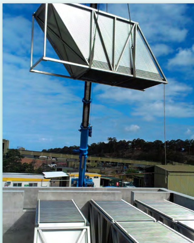
INSTALLATION OF PLATES AT CENTENNIAL MINE WTP
