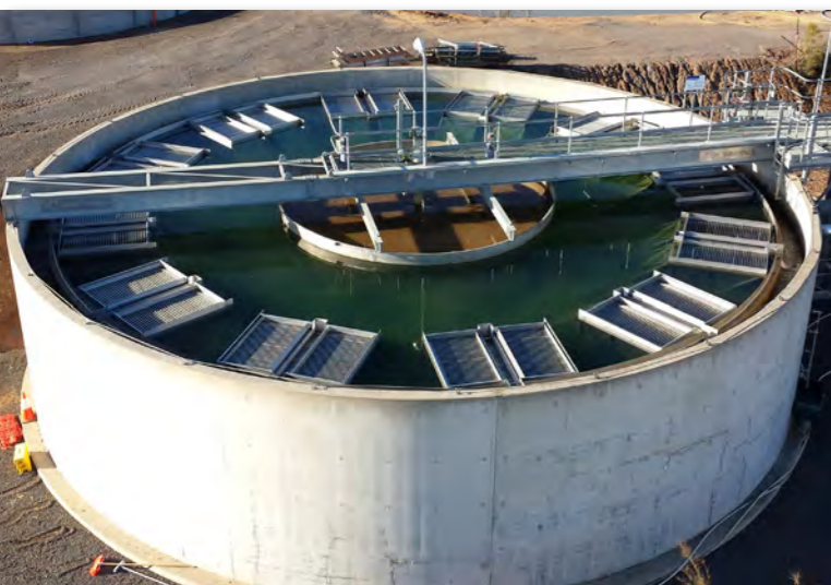
SANDHURST WATER TREATMENT PLANT
