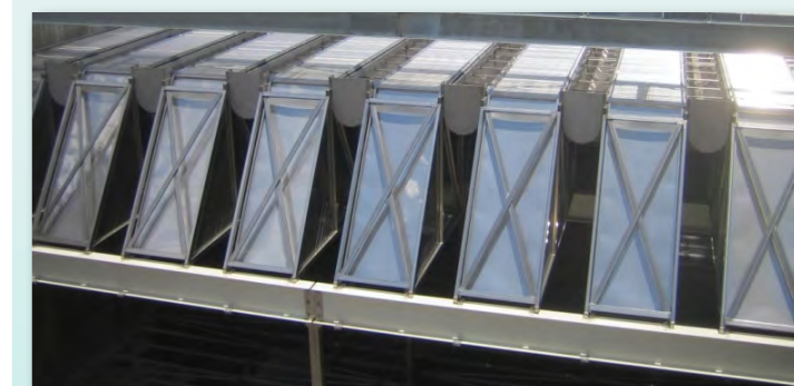
BUNDAMBA WTP (PRE-TREATMENT SEDIMENTATION)
